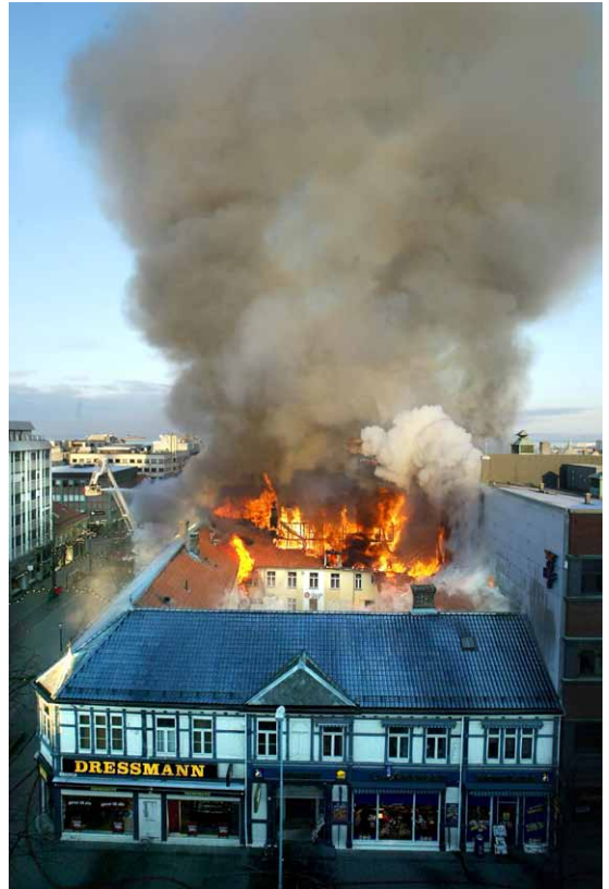
Fig. 1. The fire in the centre of Trondheim on 7 December 2002. The fire spread to engulf the wooden building in the foreground at the southern end of the fire site. The buildings destroyed by the fire were built in the 1740s and were typical of the building style of the period, although the large shop windows were of later date. Photo: Rune Petter Ness, Adresseavisen 9.12.2002. Published with permission.
